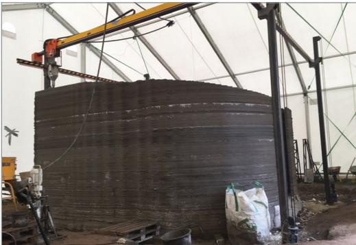
**FIGURE 2.10** – The finished 3D printed walls of the building on demand (BOD) building. 3DPrinthuset.
